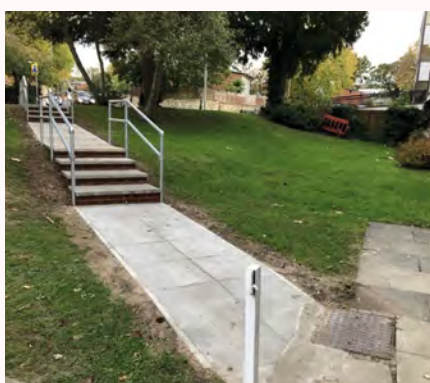
After the path improvement
