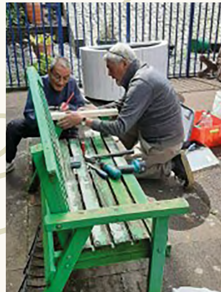
Repairing outdoor seating
